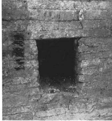
Fig. 192 a . S. Pietro in Vincoli, North clerestorey, beam hole for aisle roof, church B
